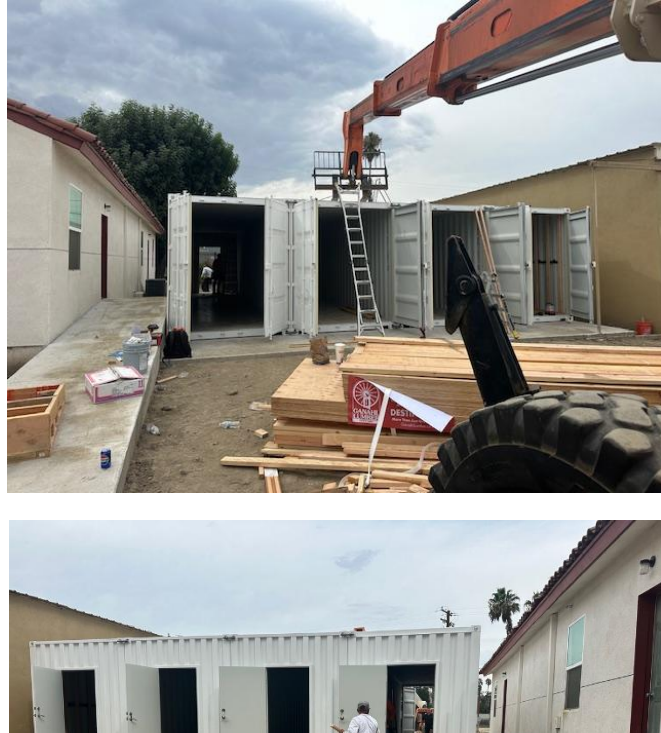
(Left) The newly poured slab. (Top R) Placing containers. (Bottom R) Container entrances, looking northeast.
