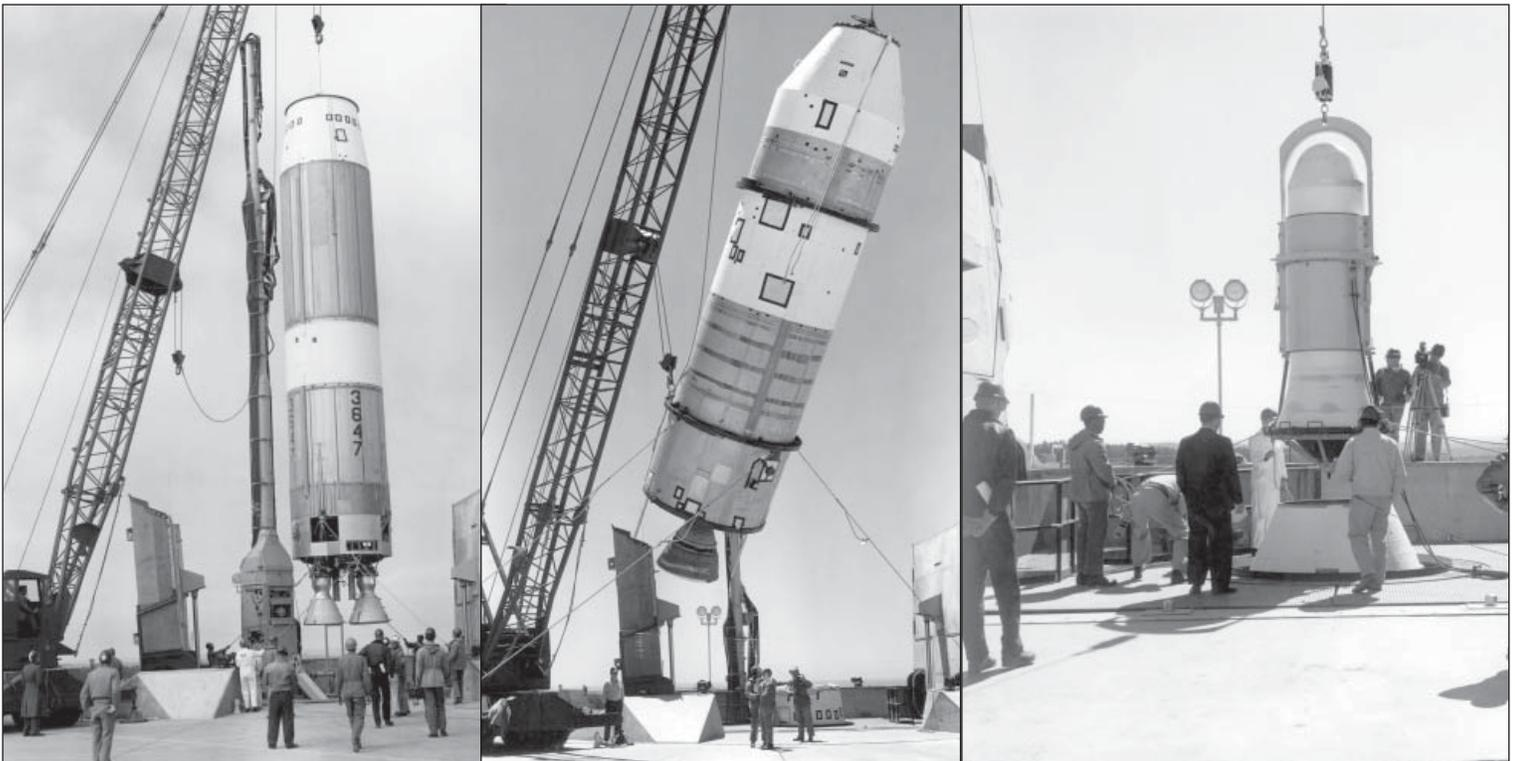
LEFT: Installation of a Titan’s first stage into the TF-1 missile silo. (USAF photo) CENTER: Installation of a Titan’s second stage into the missile silo. (USAF photo) RIGHT: Placement of the re-entry vehicle onto the missile. The author is in the foreground at the far left in the photo. (USAF photo)
